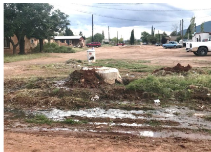
Sewage Overflow in Both Nacos (Ambos Nacos) October 2018
