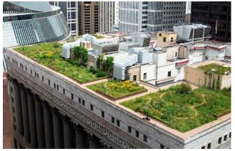
Figure 7.7. Green roof on the Chicago City Hall, a highly visible example of a public building showcasing heat mitigation (U.S. Department of State)
