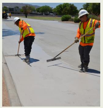
Figure 4.7. Workers applying a cool surface coating to streets in the City of Phoenix as part of a pilot project being evaluated by Arizona State University (City of Phoenix)
