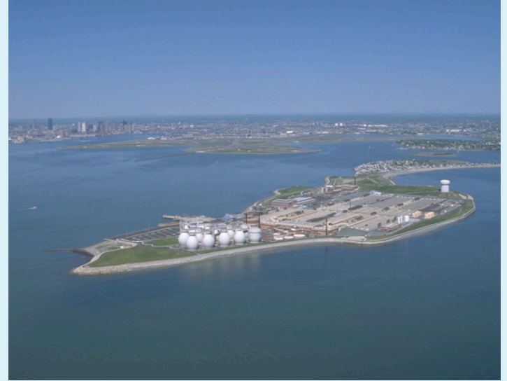
Figure: Deer Island Sewage Treatment Plant. Image courtesy of Massachusetts Water Resources Authority.
